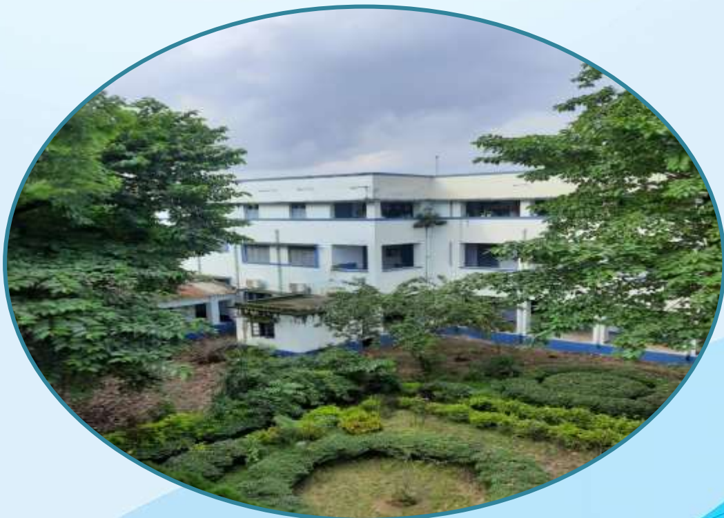
Panoramic view of College building
